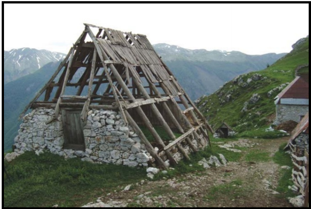
Figure 18: Some of the remainings of the old village architecture, showing the structure of the building itself, village Lukomira, Bjelašnica.
